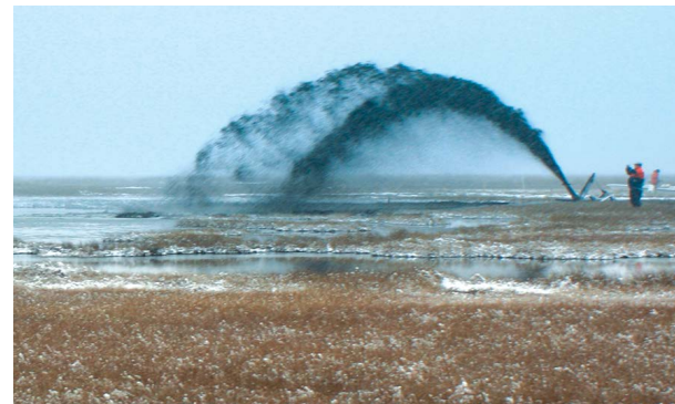
Thin-layer placement of sediment at Avalon, NJ.
